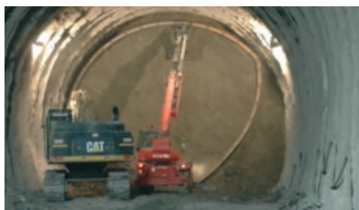
MRT 2150 placing a 2000kg (4400lbs) beam
