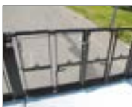
Self-closing front door with opening sensors
